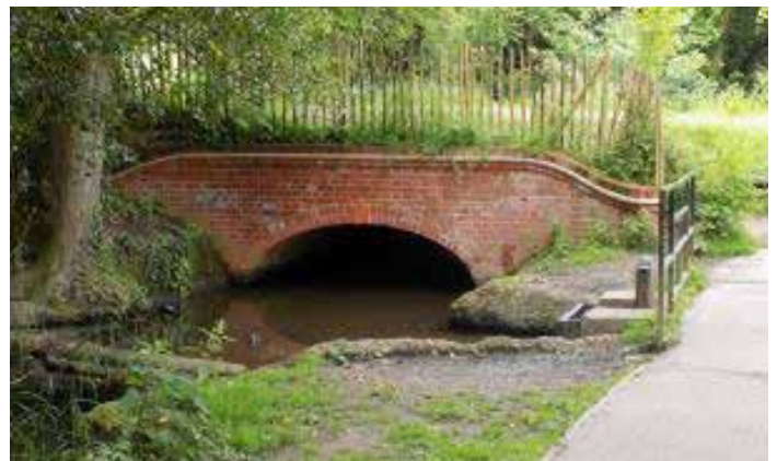
Small Pulham Bridge
